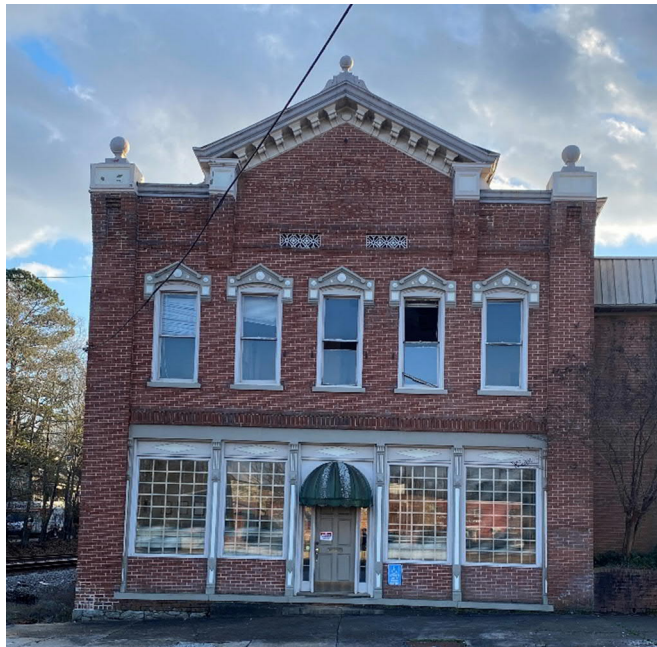
Figure 1: Historic Façade at 57 East Broad Street
